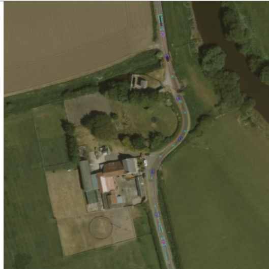
Plate 2-4: Oak Lane - Blind Corner
