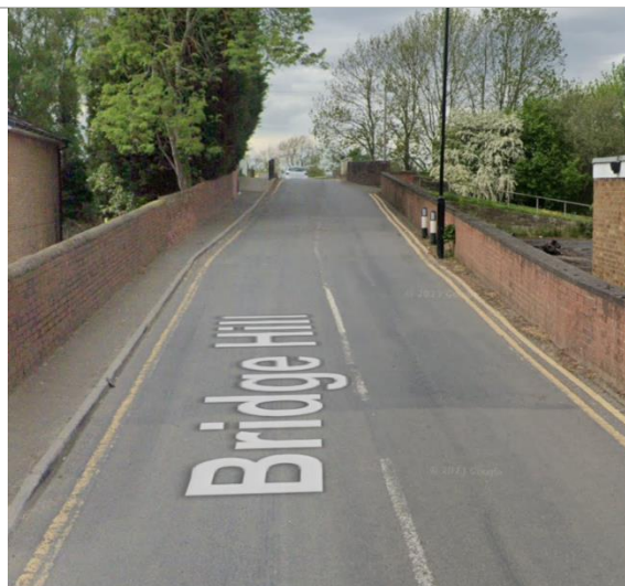
Plate 2-16: Steep Vertical Gradient on Approach to Bridge Structure
