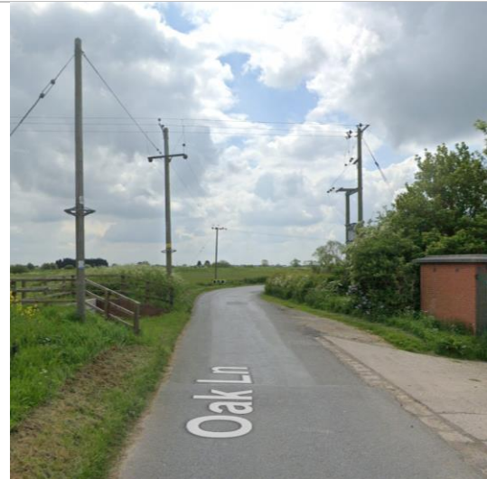
Plate 2-5: Oak Lane - Blind Corner
