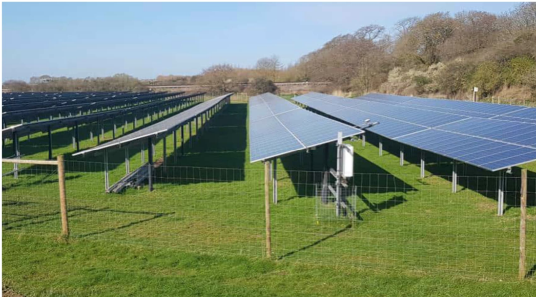
Plate 2: Example South Facing Solar PV Panels
