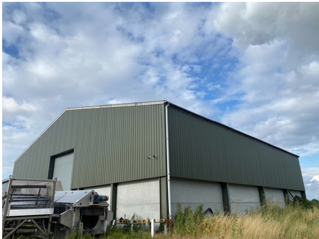
Plate 2-7: Existing Barn within Field NW08 of the Solar PV Site
